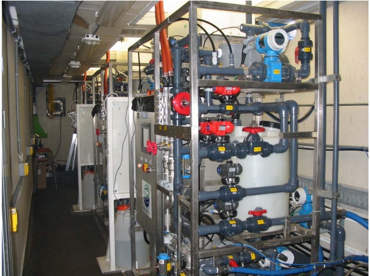
Pilot Scale Membrane-based Wastewater Treatment System
